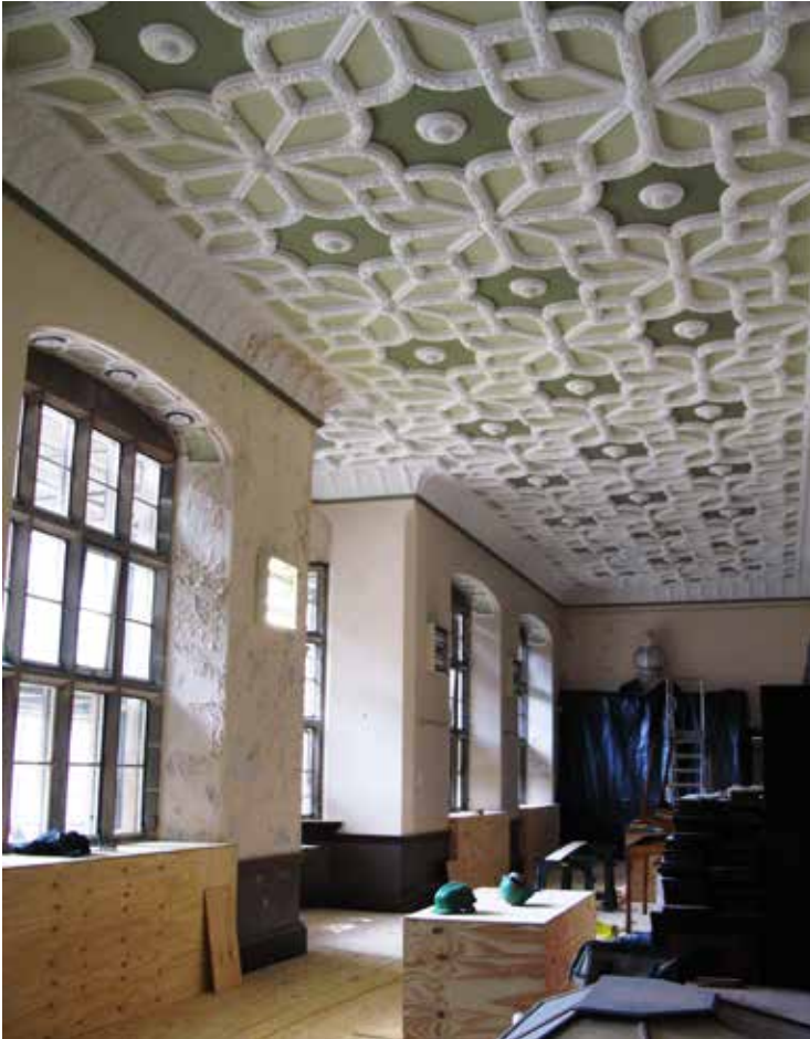
Arundell Library during renovation
