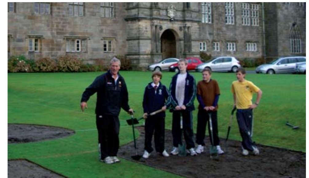
Construction of 'Rosary Garden' at Stonyhurst
